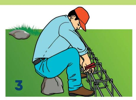
Prepare the capping beam with 3/8" rods.
