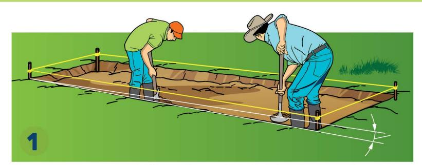
Dig a hole big enough to fit the filter, which is 4.5 metres long by 80 centimetres wide and 75 centimetres tall. The filter needs to have a 5% slope towards the outlet.
